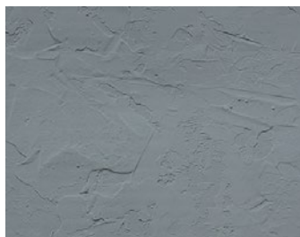
Rivestimento esterno in malta con finitura laccato opaco / External mortar coating with matte lacquered finish
