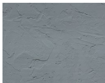
Rivestimento esterno in malta con finitura laccato opaco / External mortar coating with matte lacquered finish
